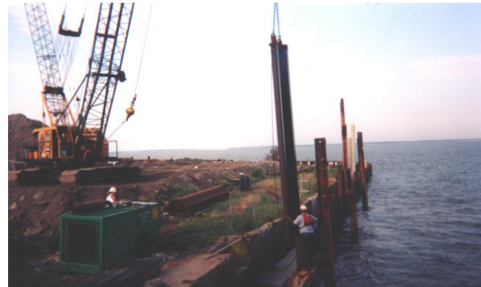
Standing steel sheet-piles for driving
