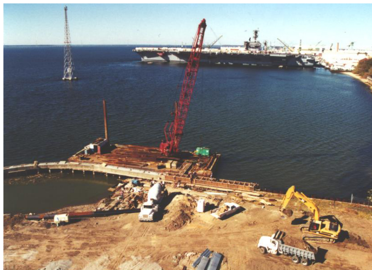
New steel sheet-pile bulkhead with concrete cap
