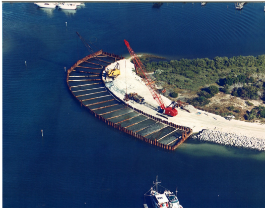
Temporary bulkhead for permanent rip-rap protection
