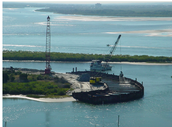
Temporary steel sheet-pile bulkhead
