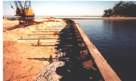
Steel sheet-pile bulkhead tie-back system
