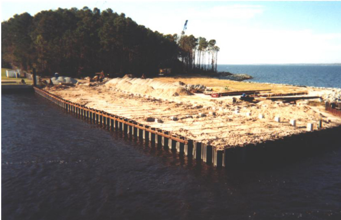
New steel sheet-pile bulkhead
