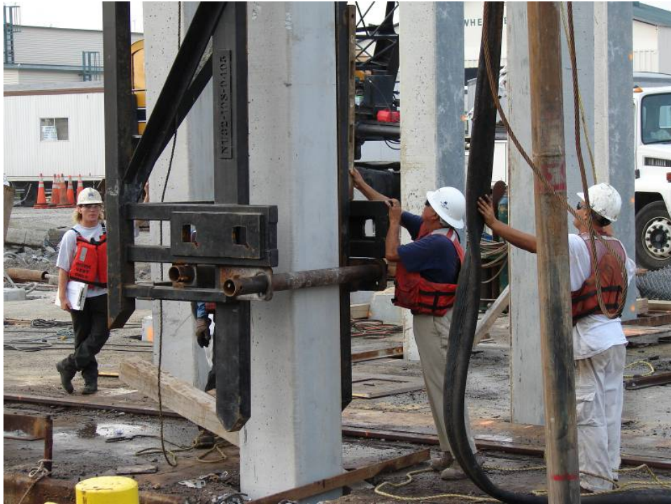
Installation of concrete piles through the existing pier deck surface.
