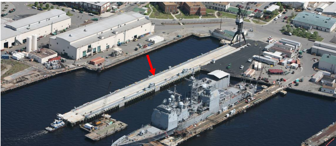
Completion of the new elevated Pier 3 structure.
