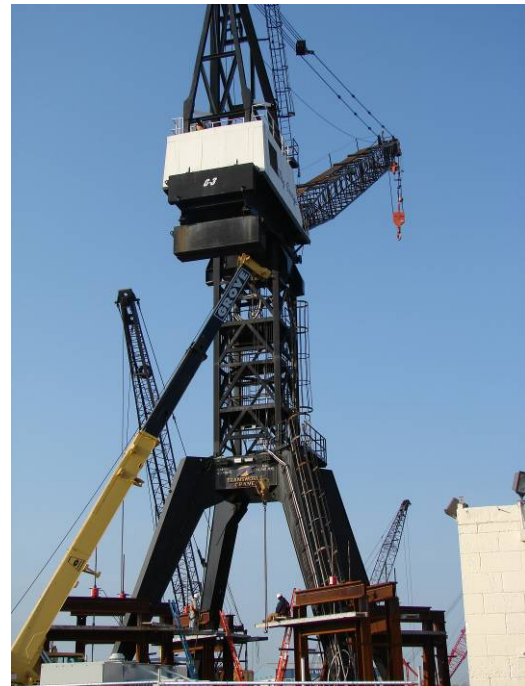
Jacking frame used to raise the portal crane.
