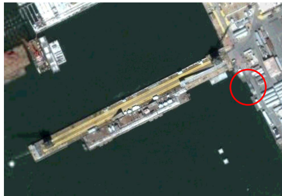
Aerial View of Pier 2 – Bulbous Bow Extension Circled
