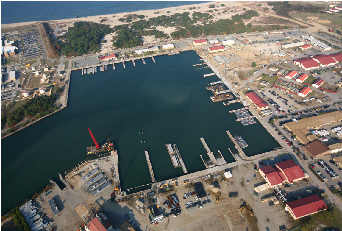
Aerial view of the project work area
