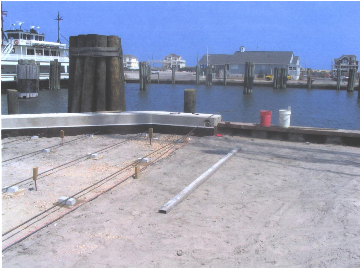
New steel sheet-pile bulkhead with concrete cap
