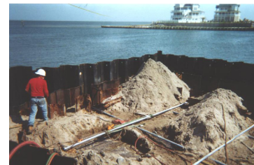
Setting the tieback system
